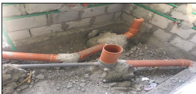
Figure 3. Modified Plumbing System Inside the Bathroom
