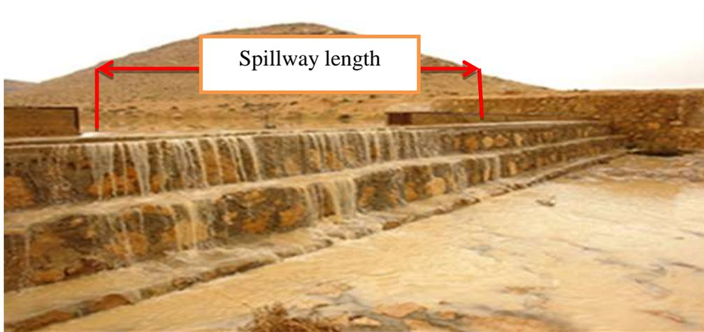
**Figure (3):** Spillway of the dyke
