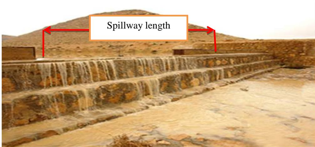
**Figure (3):** Spillway of the dyke
