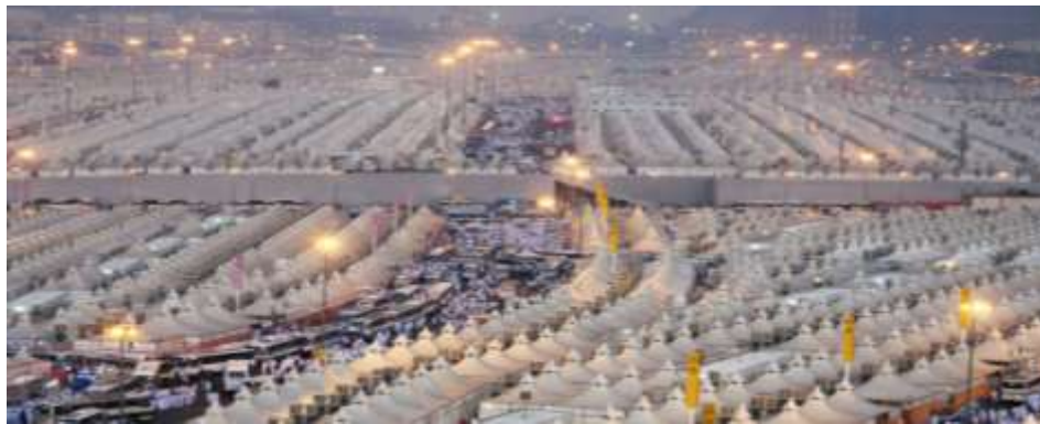
Fig.(4): Tents prepared in mina for pilgrims’ accommodation with A/C units, (Researcher).
