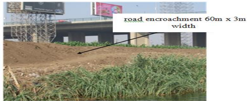
Figure(1): Citizens encroachment on the river floodplain
